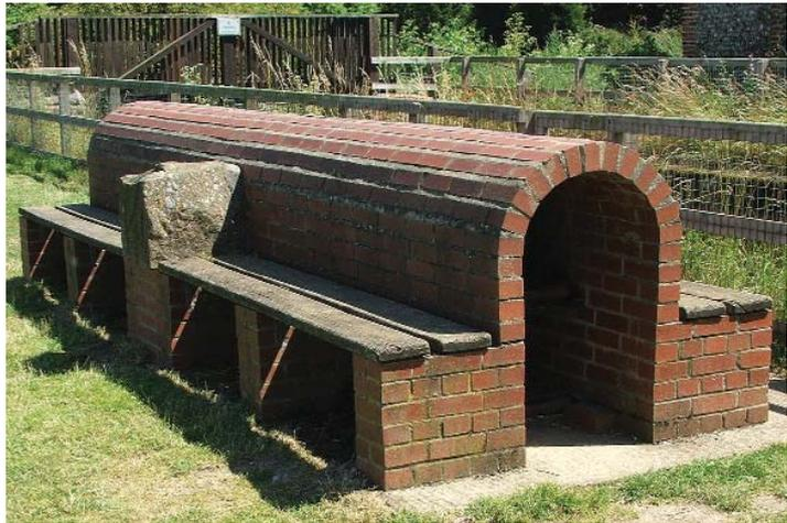
**DUAL FUNCTION:** Beside Bosmere Lock this stop plank store was built with a dual function that also provides seating for the park alongside the lock.
