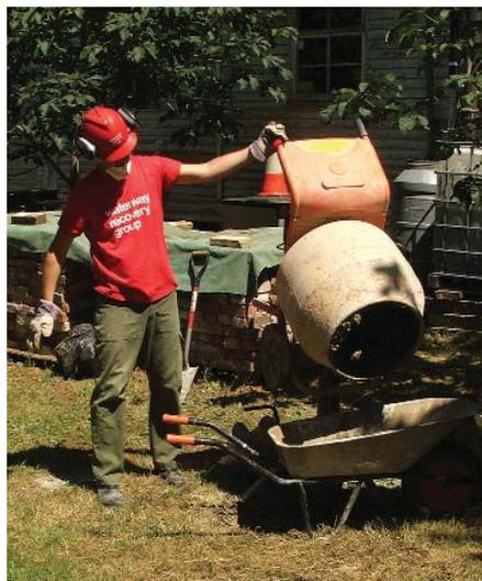
**MIXING IT:** Mixing the cement for the replacement wall. The stock of reclaimed bricks is stacked outside the large shed, used as the camps headquarters.
