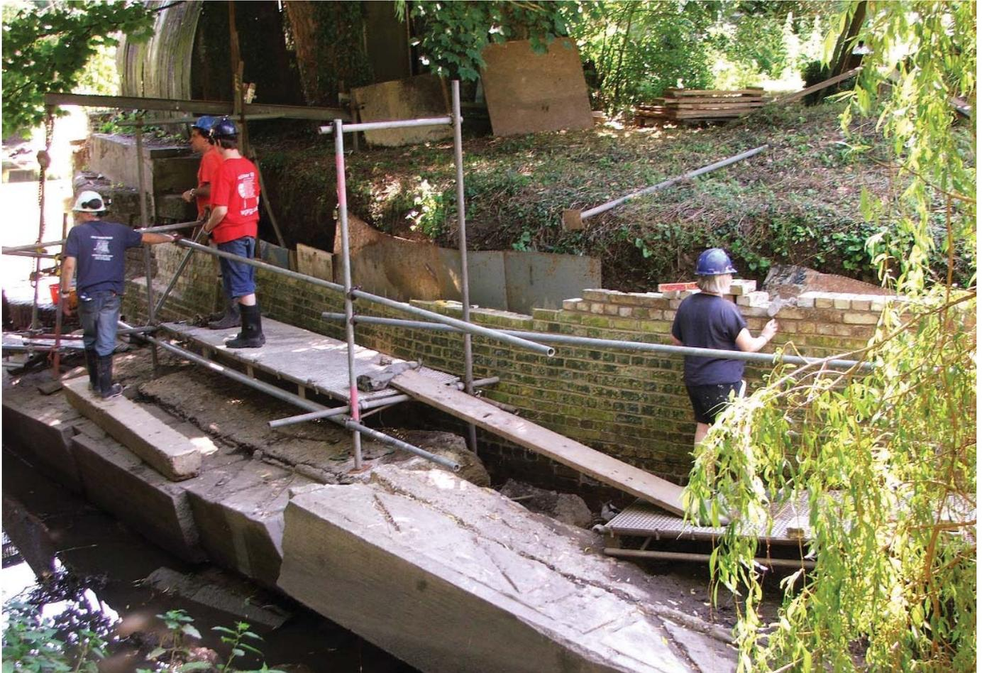
**PERMISSION:** Listed building consent was needed before the Waterways Recovery Group volunteers could work to replace the collapsed retaining wall.
